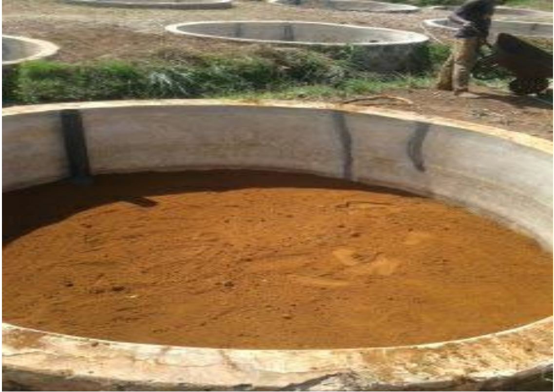
Figure 3.1 Tanks laid out with soil during preparation
