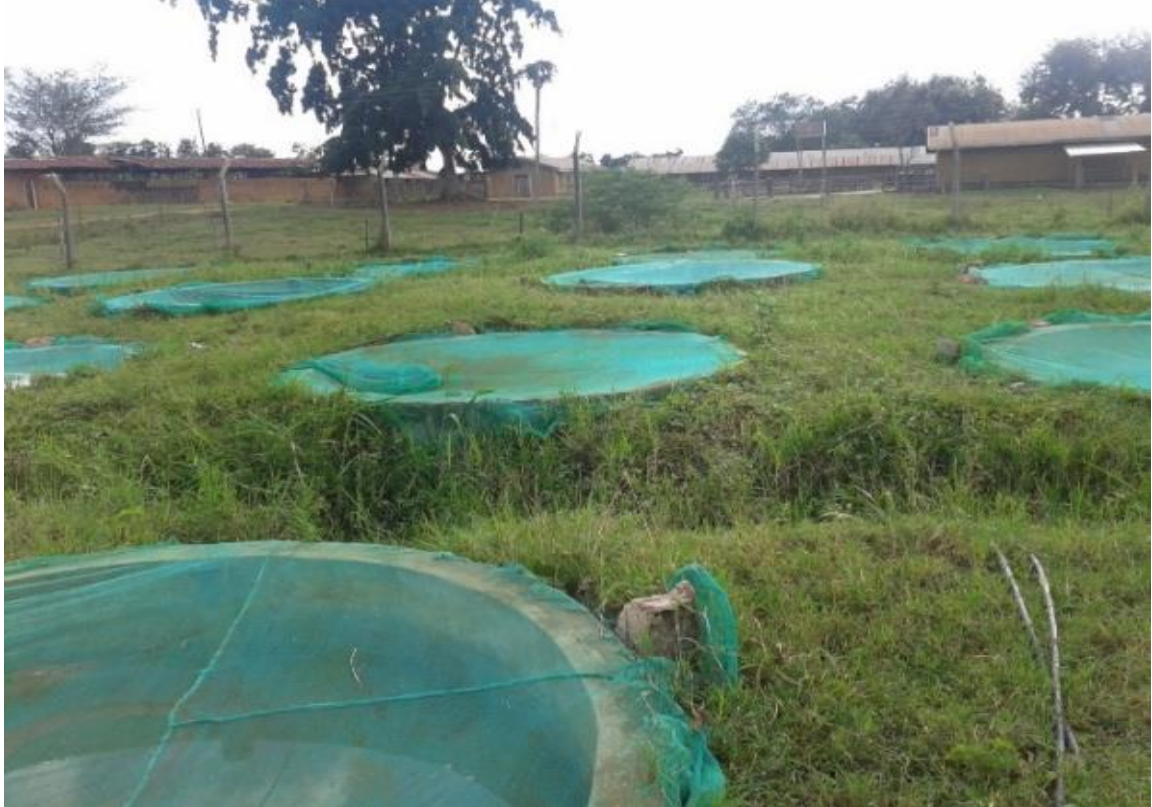
Figure 3.7 Concrete tanks covered with plastic nets
