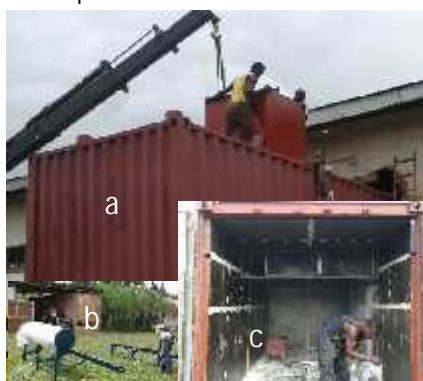
Dryer being built by local artisans: a) Installing the dryer at the project site; b) Assembling the solar system; c) working on the inside
