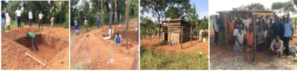
Figure 4. Farmers engaged in the construction of IMO demonstration units
