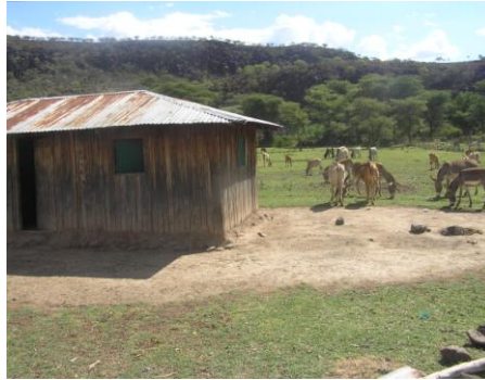
Plate 2: A photograph showing iron sheet roofed house and wooden wall house
