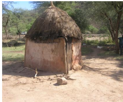
Plate 1: A typical grass thatched roof and mud walled house
