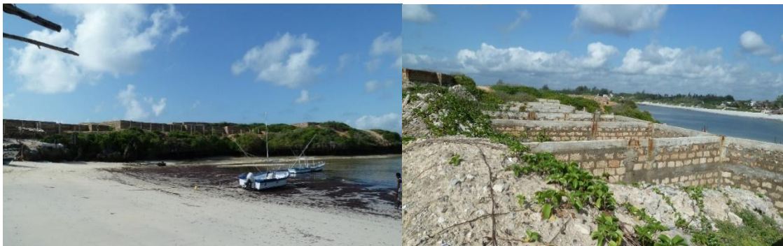
Figure 2. Illegal development on Blue lagoon headland
